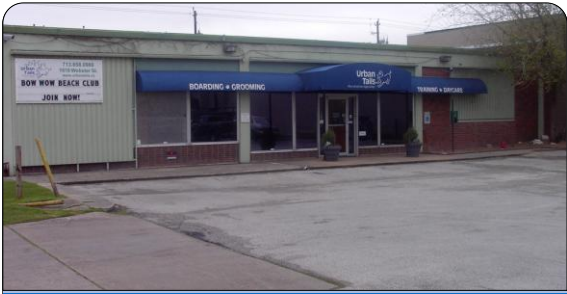
Urban Tails Building After Renovation
